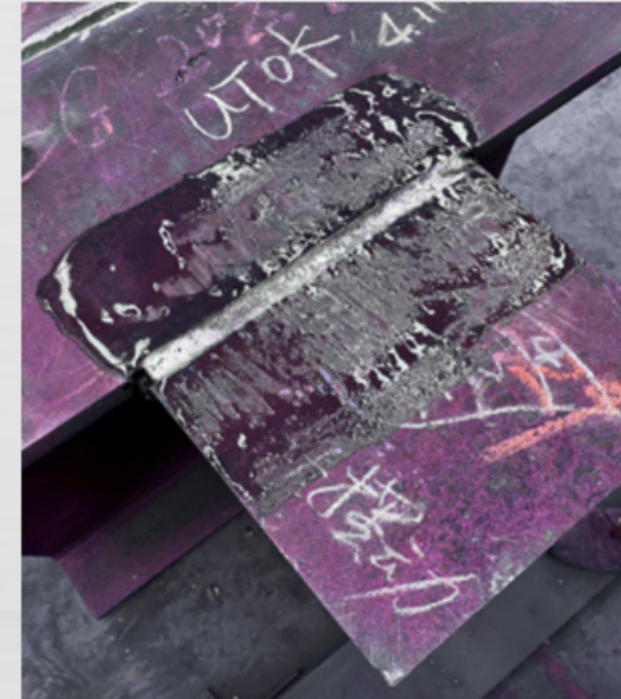
Test weld seam (UT inspection OK)
