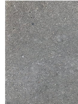
Rough concrete floor
